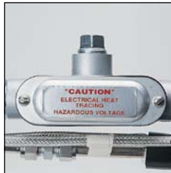
Assembled Input Power and Splice Connection Kit
