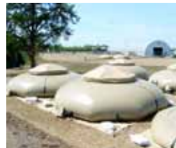
Collapsible storage tanks
