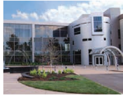
Parker Headquarters, Cleveland, Ohio, USA
